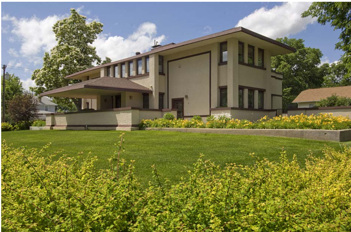
An example of his earlier prairie style design, Frank Lloyd Wright's Sutton House in McCook is one of few homes west of the Mississippi designed by the famous architect. Photo Courtesy of Nebraska Tourism.
